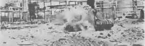
WITH A shove on the detonator, which sets up a high voltage current to a dynamite cap, top photo, M. Hazel explodes the charge. Off goes the dynamite bottom photo, which destroys the concrete block.
